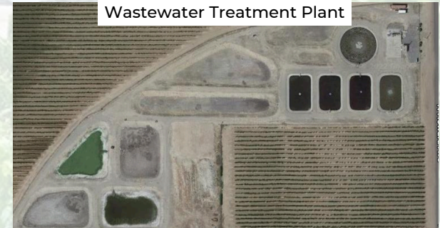
Wastewater Treatment Plant
